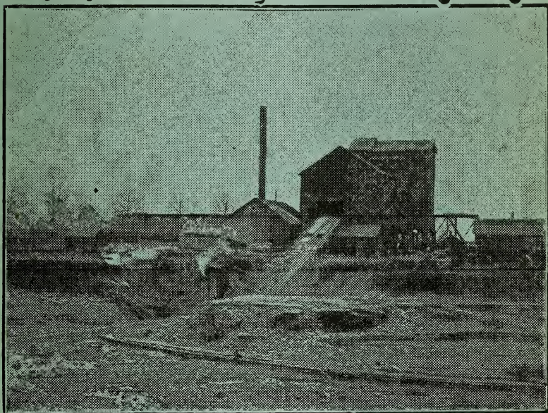
RIDGEVILLE STONE CRUSHING PLANT.
